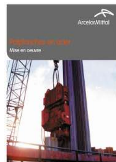
Installation of sheet piles GB, DE, FR
